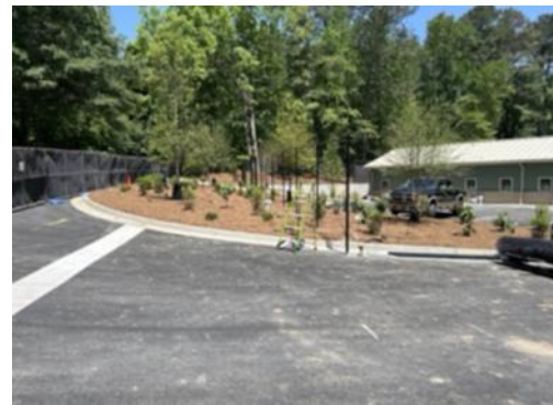
Brook Run Maintenance Facility
