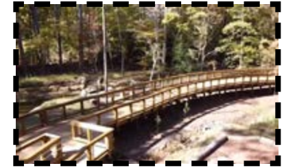
Grand Opening New DNC Boardwalk
